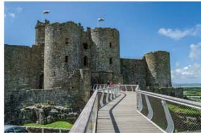
1. Examples of viewing platform and walkway in historic setting demonstrating the use of contemporary materials in order to allow the new intervention to visually contrast with the historic fabric of the adjacent structures
