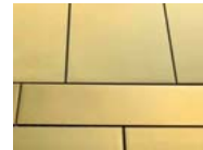
4. External Wall & Panels: Zinc Cladding: eZinc Rainbow pre-weathered zinc Colour: Gold / Grey or similar and approved.
