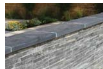
8. Parapet: Slate/Granite coping stone surround to edge of parapet. Colour to match local vernacular.
