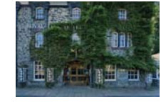
3: Living Wall: Plants to be specified and suitable for wet conditions. Plant species to be determined.
