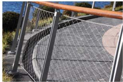
2. Example of woven metal mesh balustrade proposed to lower the visual impact of the structure
