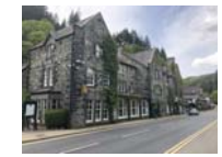
2: External Wall: Random Coursed Field Stone, to match surrounding area and Royal Oak hotel shown (shown above).
