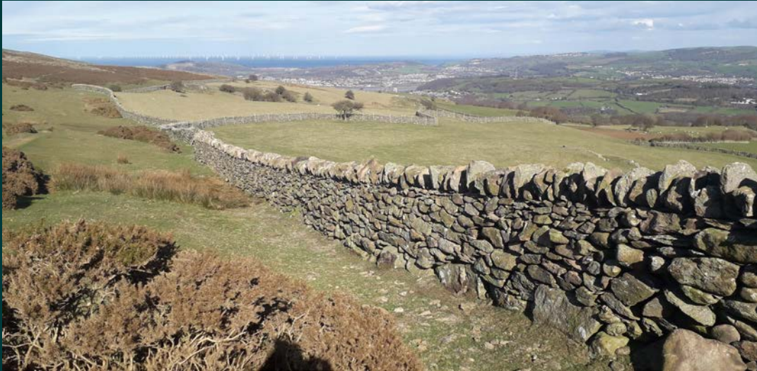
Repairing drystone walls using third party grants © SNPA
