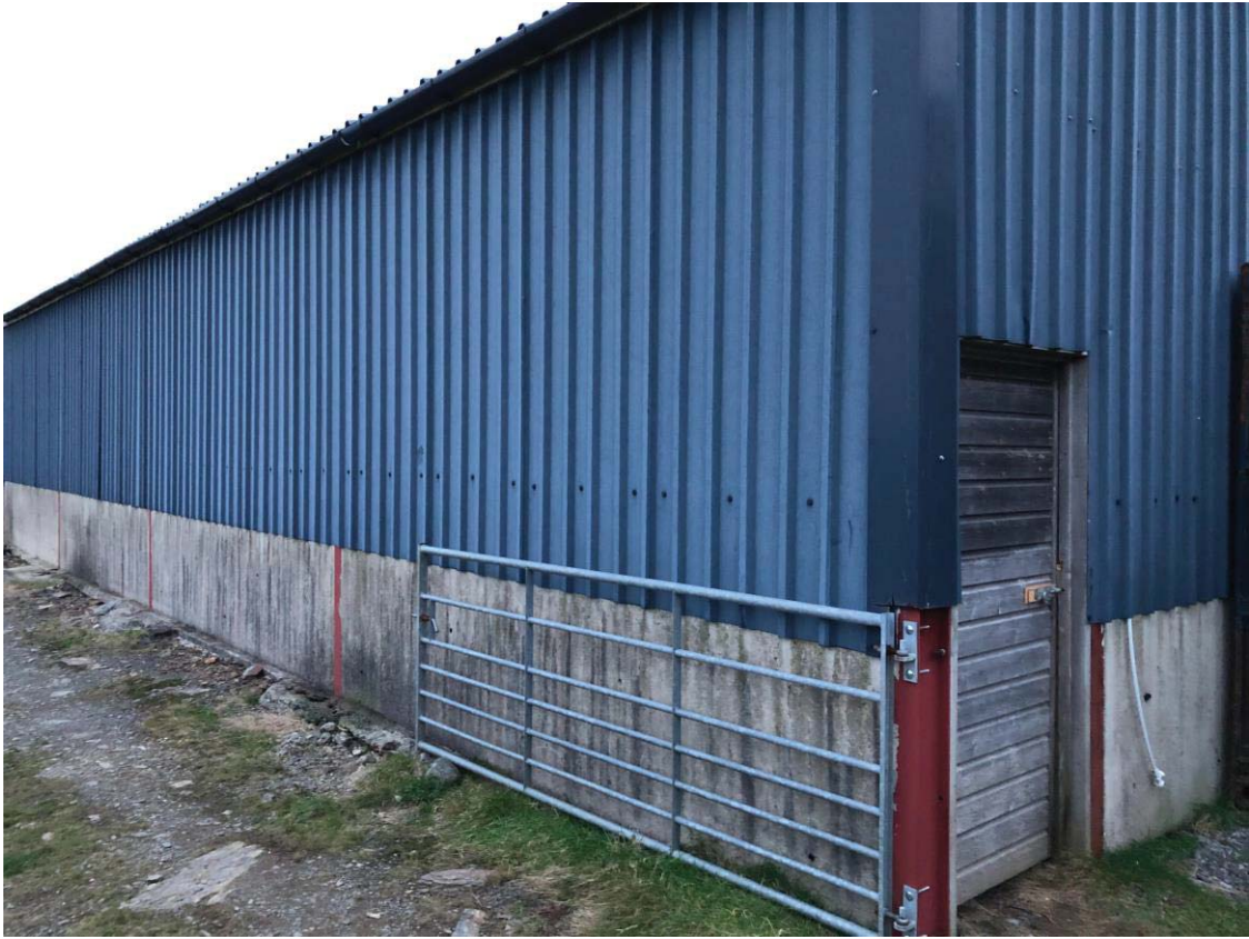
PHOTO 3: SOUTH AND PART OF EAST ELEVATION
