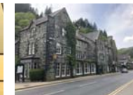
5: External Wall: Random Coursed Field Stone, to match surrounding area and Royal Oak hotel shown (shown above).
