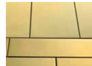
4 External Wall & Panels: Zinc Cladding: eZinc Rainbow pre-weathered zinc Colour: Gold / Grey or similar and approved.
