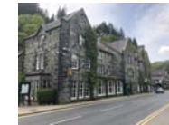
2 External Wall: Random Coursed Field Stone, to match surrounding area and Royal Oak hotel shown above.
