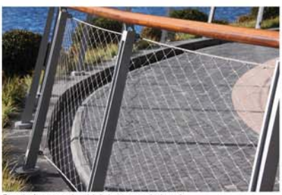
2. Example of woven metal mesh balustrade proposed to lower the visual impact of the structure
