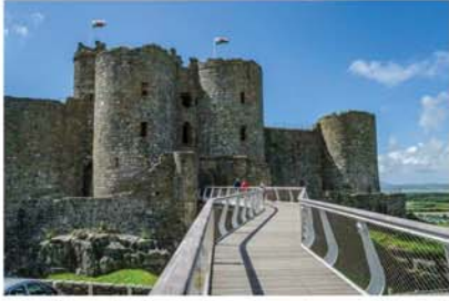
2. Example of woven metal mesh balustrade proposed to lower the visual impact of the structure
