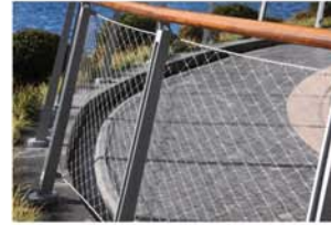
Example of woven metal mesh balustrade similar to proposed
