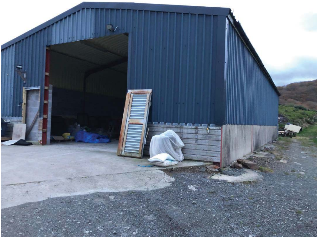
PHOTO 2: WEST AND SOUTH ELEVATION
