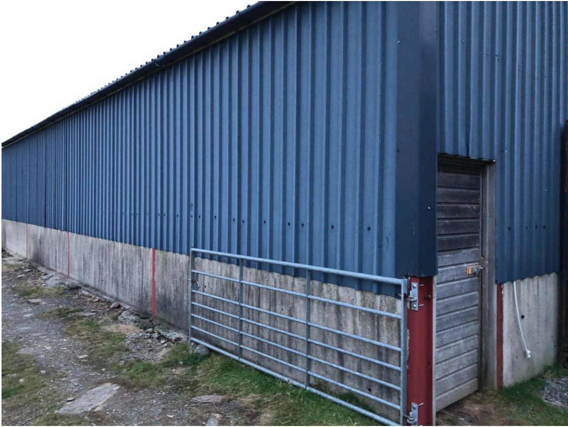
PHOTO 3: SOUTH AND PART OF EAST ELEVATION
