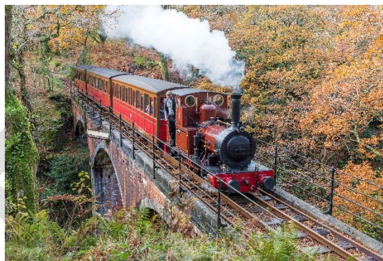
Tallylyn Railway crossing Dolgoch viaduct (Component Part 6) © Rheilffordd Tallylyn Railway
