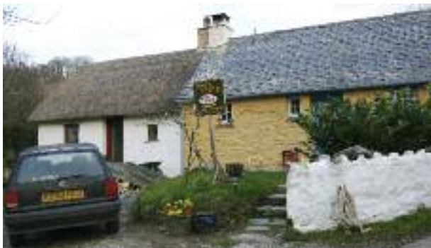
Re-use of existing building combined with use of traditional clom walled and thatch roof extension
