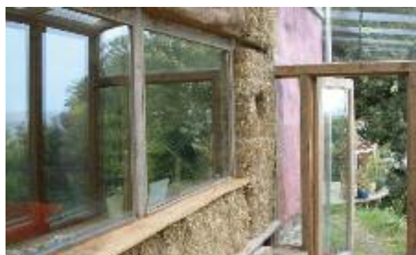
Straw bale and local timber: fresh uses for the 21st Century
