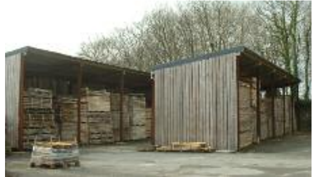
The use of locally produced low-impact materials and new techniques may produce appropriate contemporary buildings (Coed Cymru wood store, Pembrokeshire)
