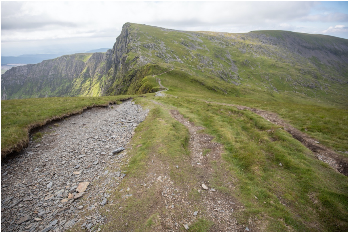
Widening footpath and erosion along Craig Cau (P12 on map in figure 2).
