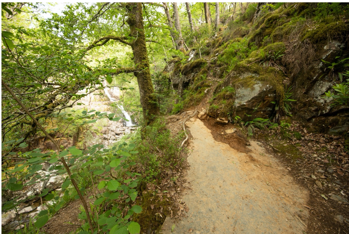
Erosion of the river bank where paths have been created and used heavily to access Pistyll Cain from the main track (point 4 on the map in figure 2).
