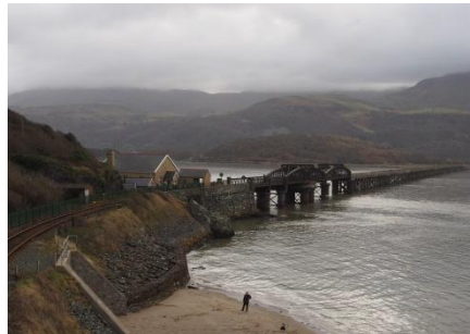
Trestle railway bridge over the Mawddach Estuary. Image © Fiona Fyfe
