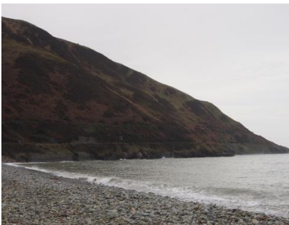
In the north of the SCA, the cliffs are so steep that the road and railway line have been cut into them. Image © Fiona Fyfe
