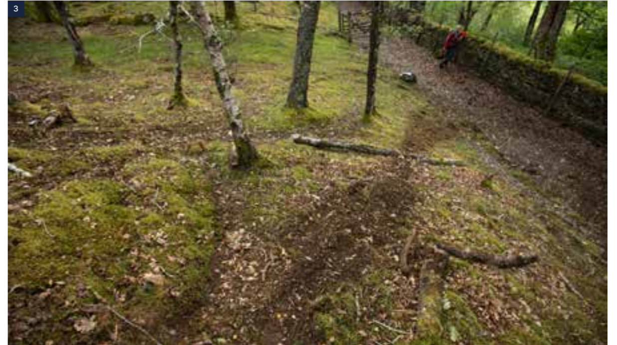
3 and 4. Motorbike damage to an area of the woodland near to the entrance to the main woodland itself at SH666391.
