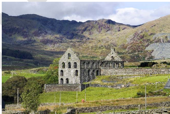
Ynyspandy Slate Slab Mill (Component Part 4) © Crown Copyright
