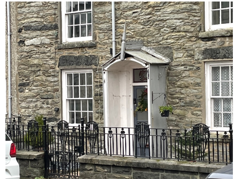
41 Rubble stone at Y Gelli, Heol Tegid. Note also the slab porch and good arts & crafts railings. (2021).
