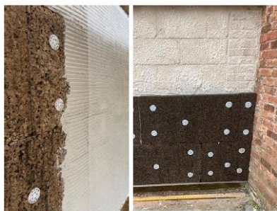
33 Application of Cork Board and render coats.
