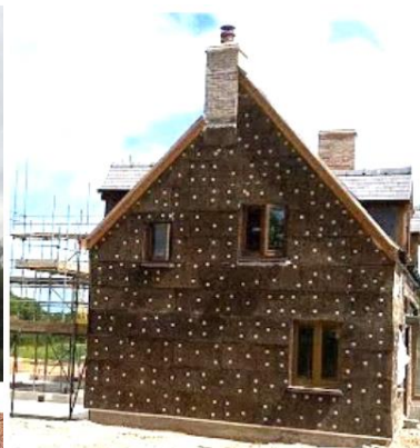
34 Cork boards installed, prior to application of render coats.
