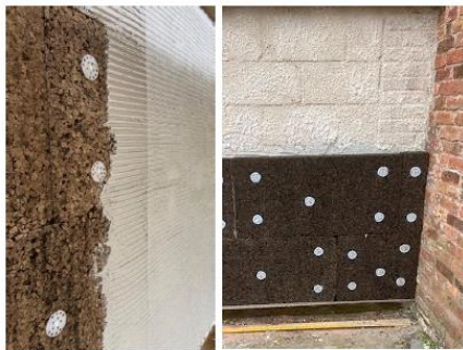
33 Application of Cork Board and render coats.
