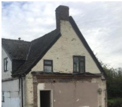
32 Typical gable following removal of a later extension.
