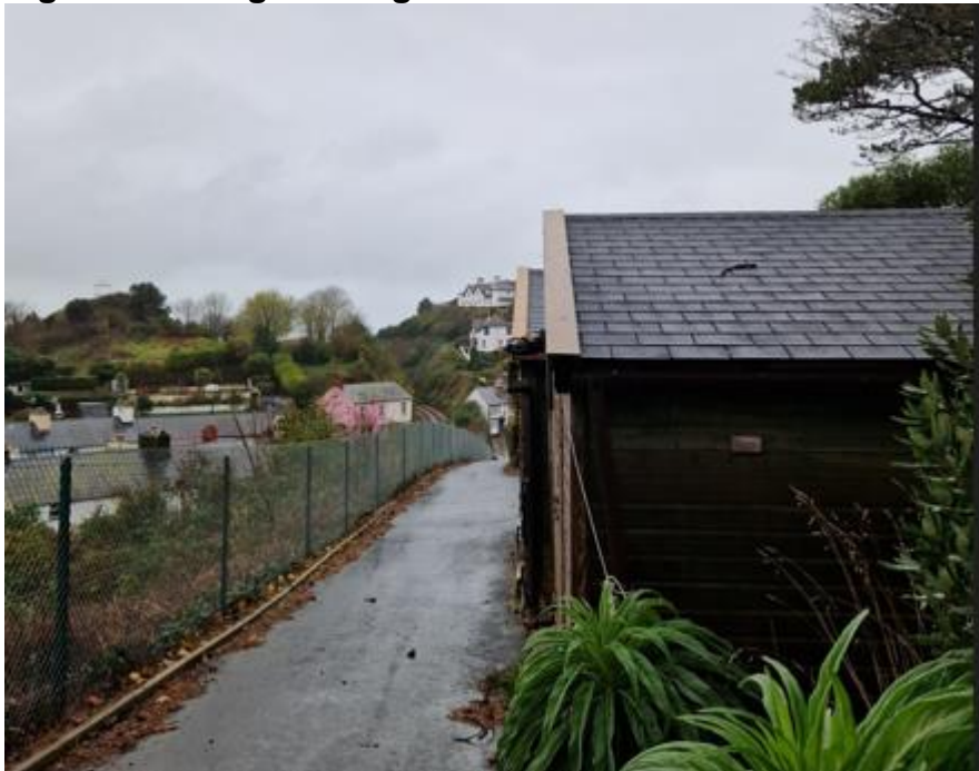
Figure 4: Garages along access lane
