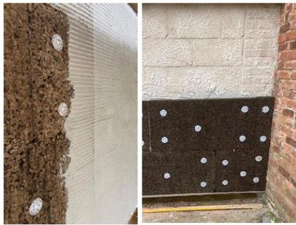
33 Application of Cork Board and render coats.
