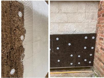
33 Application of Cork Board and render coats.
