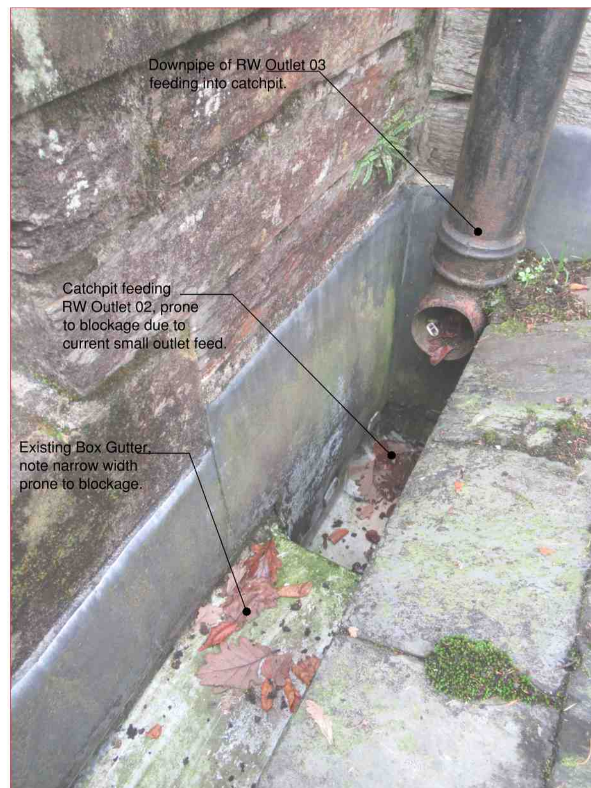
Photo of Existing of catchpit Serving RW Outlet 02 from Roof Slope R6 (Photo 5796)
