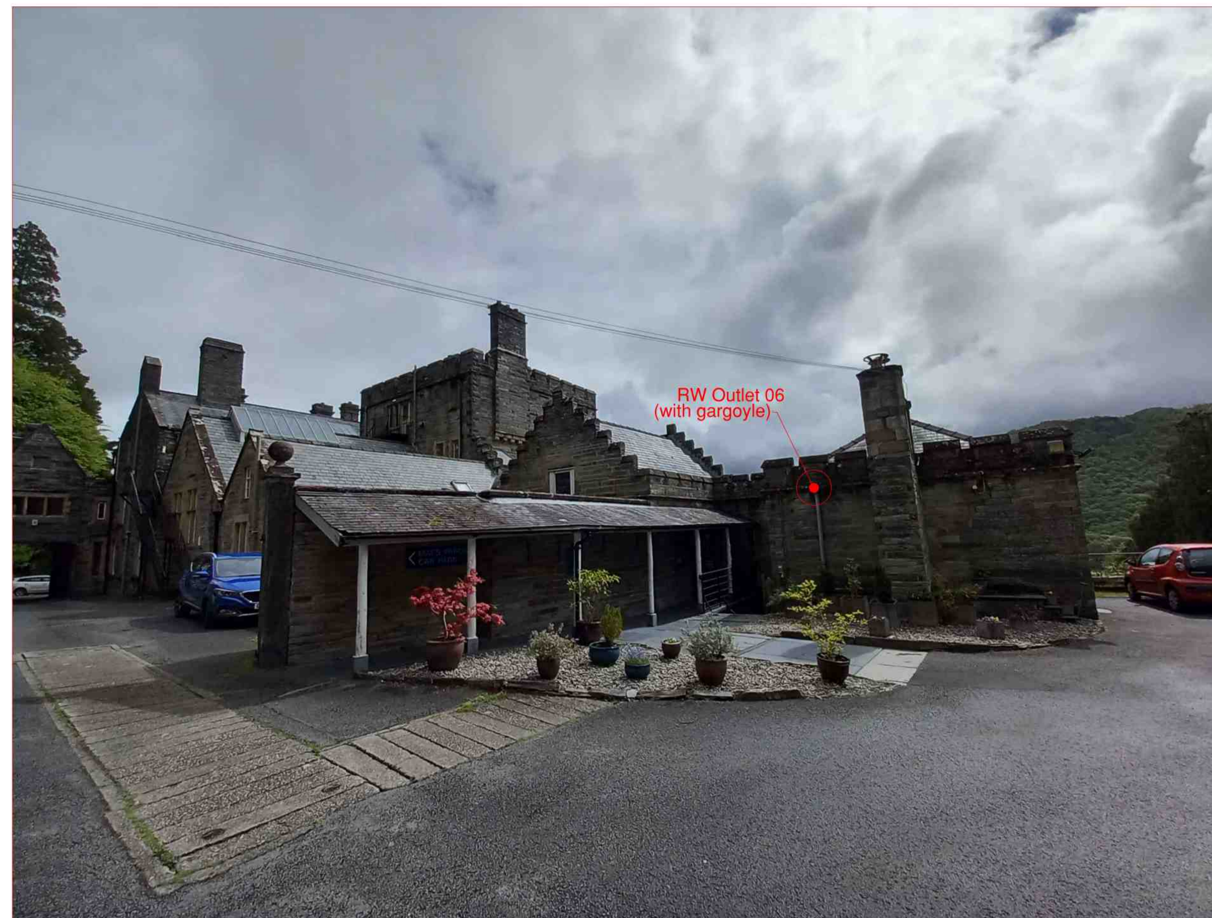
SIDE ELEVATION ELEVATION C1 (Photo 06)
