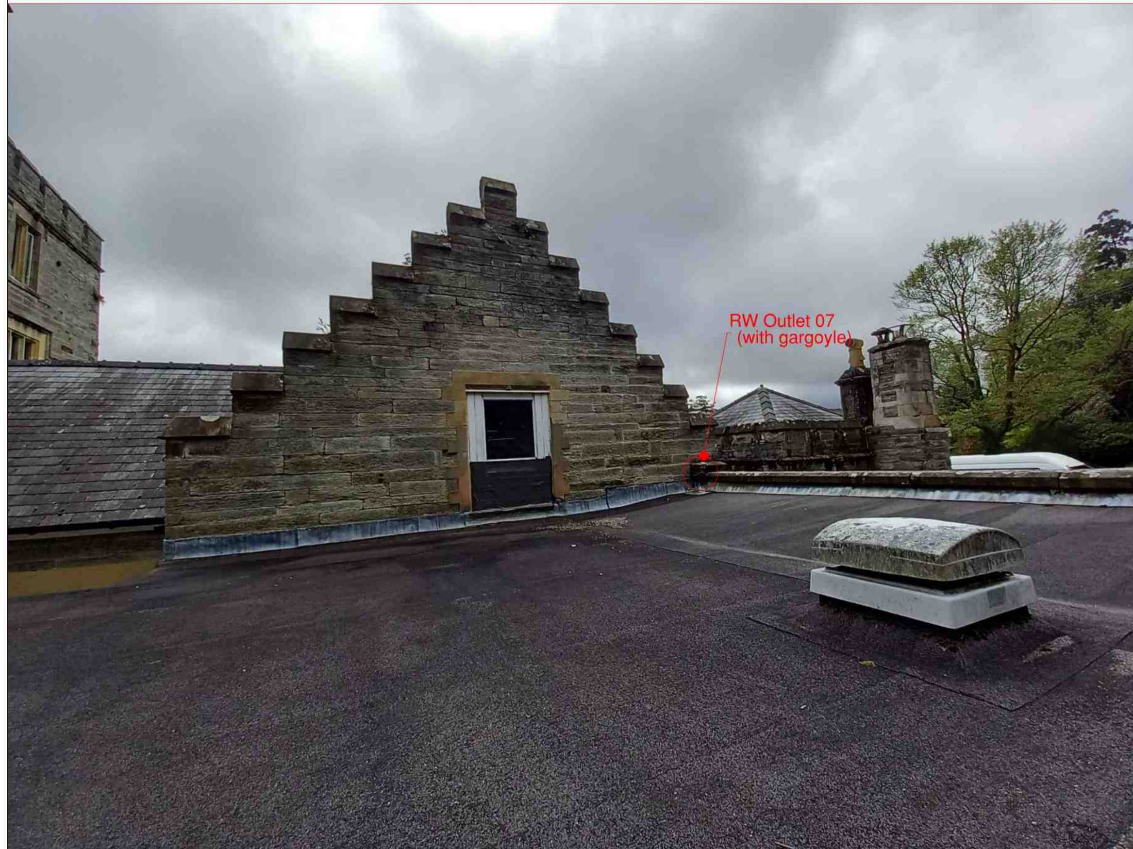
REAR ELEVATION View over Single Storey Flat Roofs) ELEVATION D1 (Photo 10)
