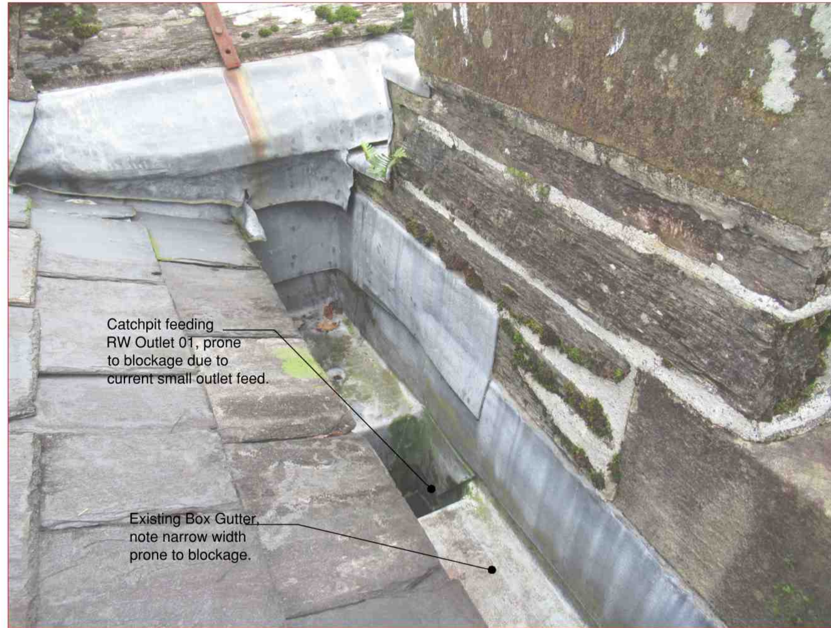
Photo of Existing Catch Pit Serving RW Outlet 01 from Roof Slope R3 (Photo 5761)
