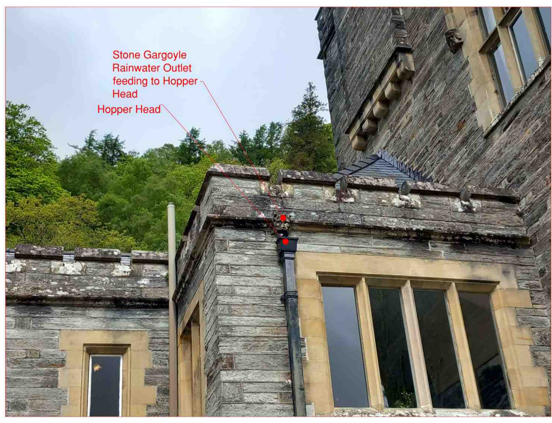
Close Up View of Rainwater Outlet with Stone Gargoyle (Photo 11)
