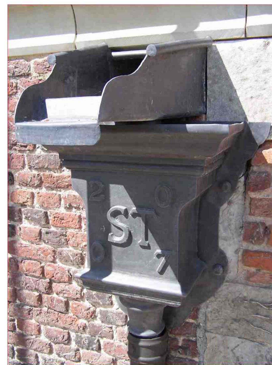
INDICATIVE PHOTO (Showing Typical Lead Chute and hopper head detail) OPTION 1 OUTLET TYPE
