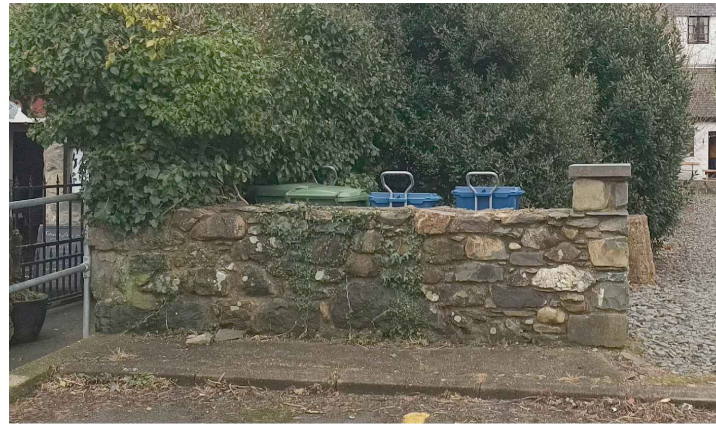
Rear Boundary Wall
