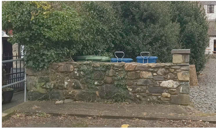
Rear Boundary Wall
