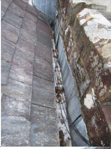
Chimney CH10. Note flue is broken at top. These flues are likely to be asbestos type flues. Any repair should take this into account. IMG\_594 4
