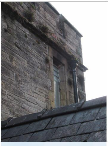
View of roof slope R12 fascia board with woodworm and some cracking at the cement flush pointing to below the kneeler that should be raked out and repointed in lime and flush pointed. Cast iron gutter requires decoration, as reported. The stonework to the gable, as can be seen at the end here, is worn.
