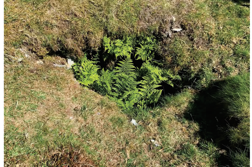
35. The opening in the ground that may be the result of settlement of backfill within a former mine shaft
