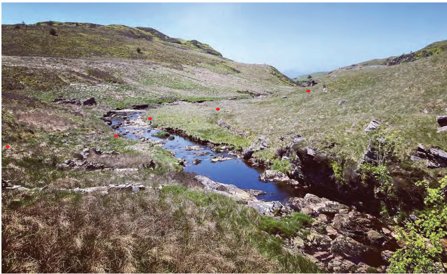
11. View west at the proposed river crossing with the pipeline extending along the north riverbank. Abstraction Point 'A' is in the middle distance, to the right of the ruined stone building.
