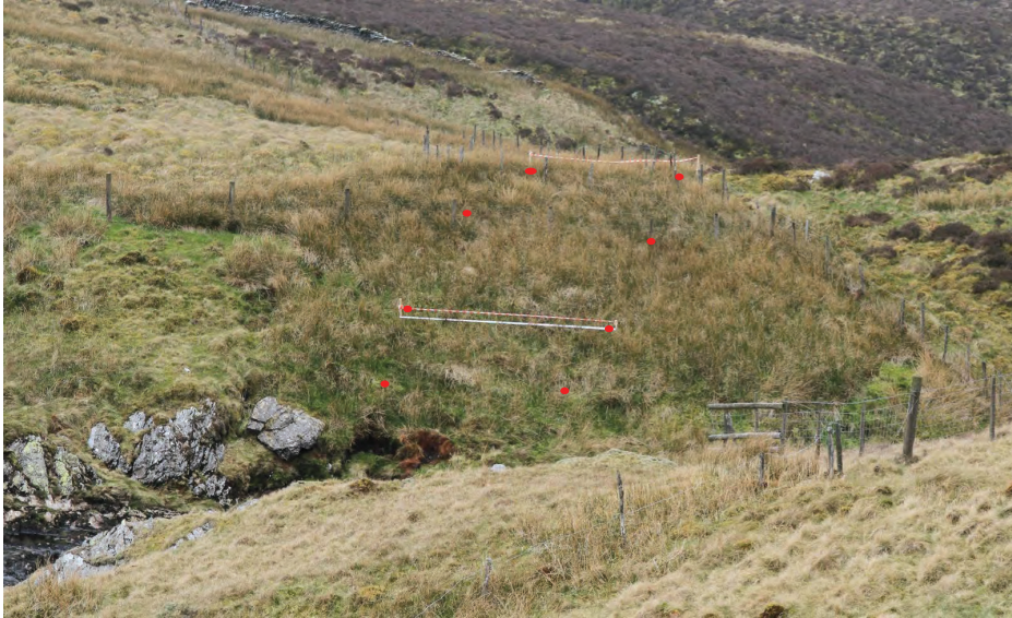
34. The location of the rock cutting looking south with the water intake and weir to be located in the foreground. The coloured ribbons and the red dots show edges of the 5m wide cutting through the crest of the hill. On completion the cutting would be backfilled and the hill soils and vegetation reinstated.
