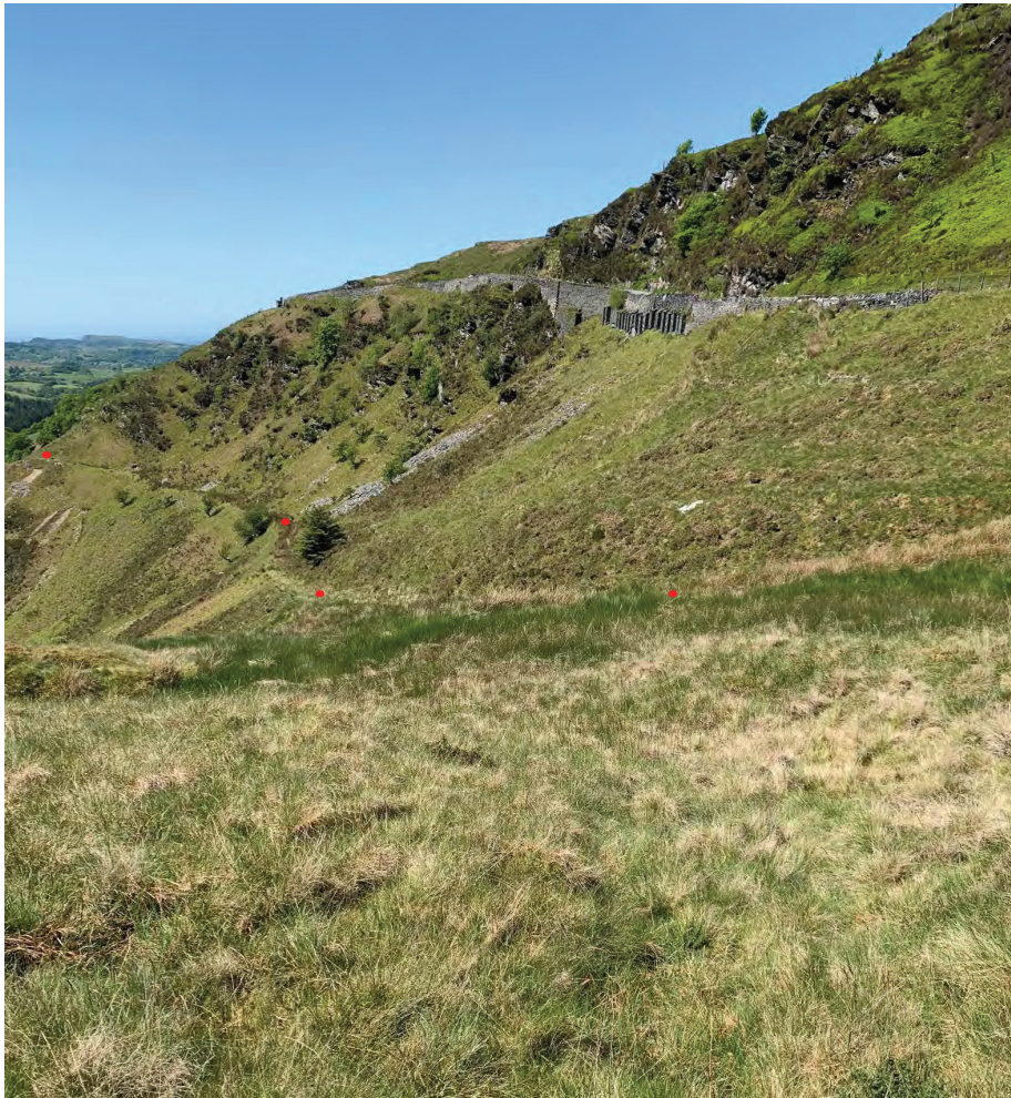
13. View west where the pipeline converges with the trackway (Footpath 22). The B4391 and its retaining structure can be seen clearly in the top right of the image. The dark green strip descending right to left across the middle of the image is a small watercourse that the pipeline must cross.
