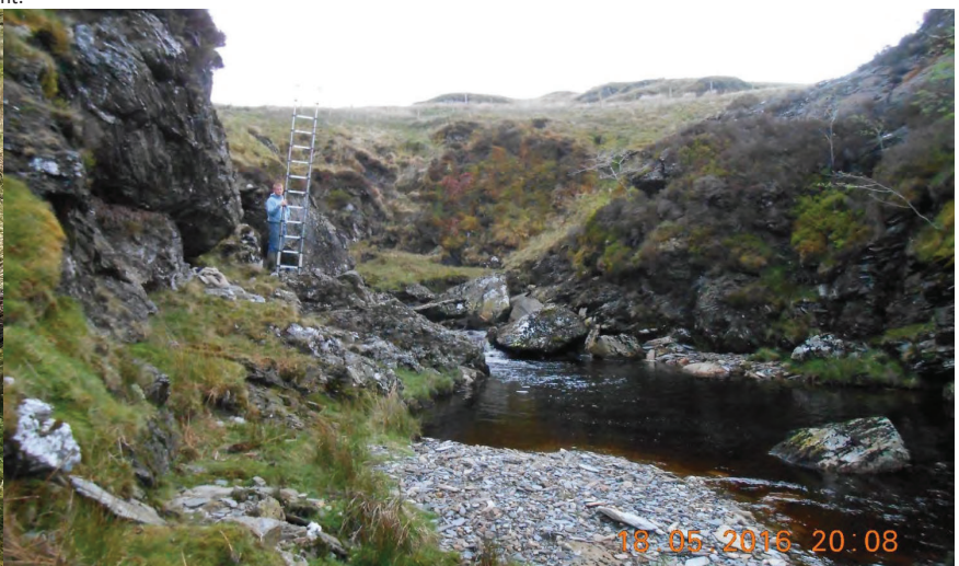
7. The river passes through a narrow gap between steep rock outcrops. This is abstraction point alternative B and would have required a weir of approximately 3.5m height.
